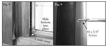
The flat side of the side rails should face the exterior, and the side with the groove should face the interior. See fig. 7, take the left side rail and slide the top of it onto the tongue of the cassette housing end cap. See fig. 8, gently slide the bottom into place on top of the crank cover at the sill. Repeat for the right side.
