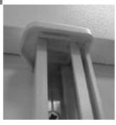
4. Fix End Caps to the top and bottom of the Rack Extrusions before fixing in place.
