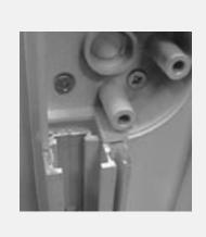
3. Cut the Rack Extrusions to fit above the Gear Housing. The Rack Extrusions run the full height of the window.
