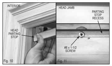
Double Check diagonal measurements. Adjust the screws as necessary to square the frame. Replace the parting stop at the head jamb of the window.
