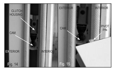
To avoid marring the frame when tilting the sash back into place, retract the latches. On the top sash, place a hand at each end, on top of the sash over the tilt latches. Slide both finger tabs toward center to retract the latches. While retracting the tilt latches rotate the top of the sash towards the exterior until it is in operating position on the jambliner. Release the finger tabs, allowing the latches to snap into place. Slide the sash to the top of the frame. Repeat for bottom sash.
