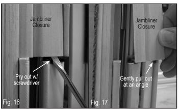
See Fig. 18 & 19. To replace the jambliner closure after finishing the interior of your window, take the leading edge of the hook leg on the jambliner closure and slide it in the grooves in the jambliners all the way up to the head jamb. Press the jambliner closure into the grooves in the jambliner, snapping it snuggly into place. Replace the head parting stop, centering it side to side. Follow the sash installation instructions on page 4 for installing both sash.
