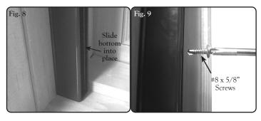
A small pile opener is included in the parts kit. Locate where the pre-drilled holes are in each side rail and place the small pile opener centered over a hole for easy access to the screw hole. See fig. 9, secure the side rail in place using the supplied #8 x 5/8" screws (G). Repeat for each screw hole on each side rail. The small pile opener is only used to separate the pile while applying the screws. Take out when all screws are installed.
