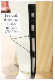
Attach sash lift Part B (clear part) to the frame. Place part B (clear part) with the open side of the screw box facing the exterior. This creates a ramp to lift the sash. Secure in place using the provided screws. Ultra/Heritage units use #8 x 1" screws and Vista-Luxe units use #8 x 3/4" screws.
