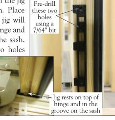
Attach Part A to the sash using the provided screws in the pre-drilled holes.
