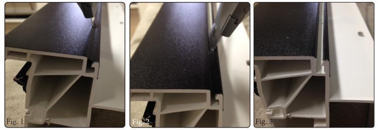
See Fig. 2. Score the other side of the accessory grove with the utility knife. Remove the small strip of foil from the frame.
