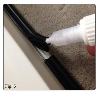
See Fig. 4 & 5. Using the black 4.8mm seal Art#864992 install the seal by pressing the house side of the seal into the top of the sash and start in the center of the sash. We want the single joint to be at the center of the sash and at the head so no water has a way in. Wrap the seal around full perimeter and cut it to length to butt it up to the other end. Use a super-glue to join the two ends together.
