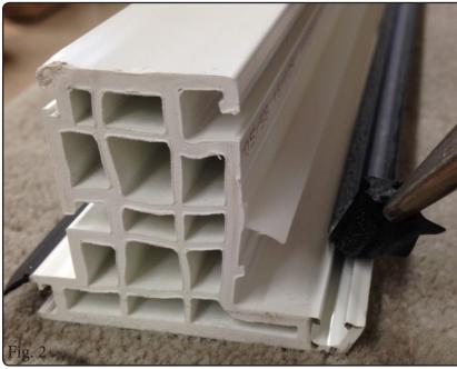
See Fig. 3. Once the seal has been removed from the sash use a rotary tool and clear out the weld spur in each corner of the sash so the new seal can be wrapped around full perimeter without any joints.
