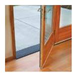
ADA-compliant sills (thermal break and non-thermal break) for swinging doors create a flush surface for easy access to pass through.
